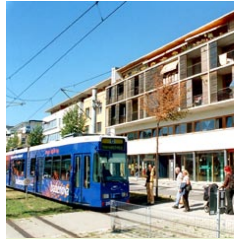
Public transport orientated development: a development form that can enable sustainable transport; high densities around public transport interchanges (Freiburg).
